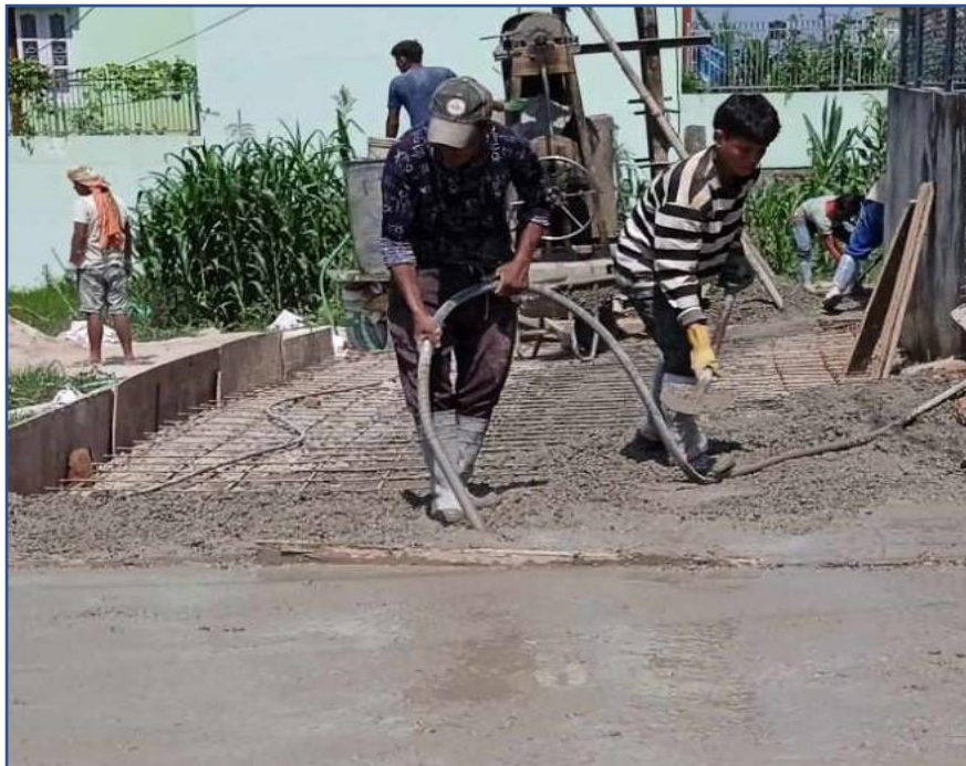
Fig : compaction by using vibrator
