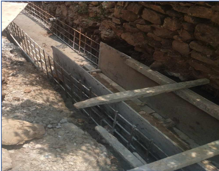
Fig : formwork placement
