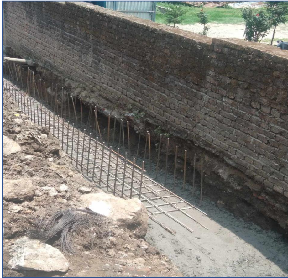
Fig : placement of re bars after PCC
