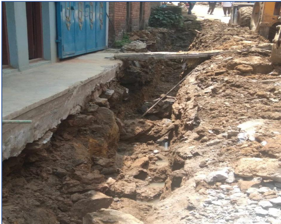
Fig: excavation works
