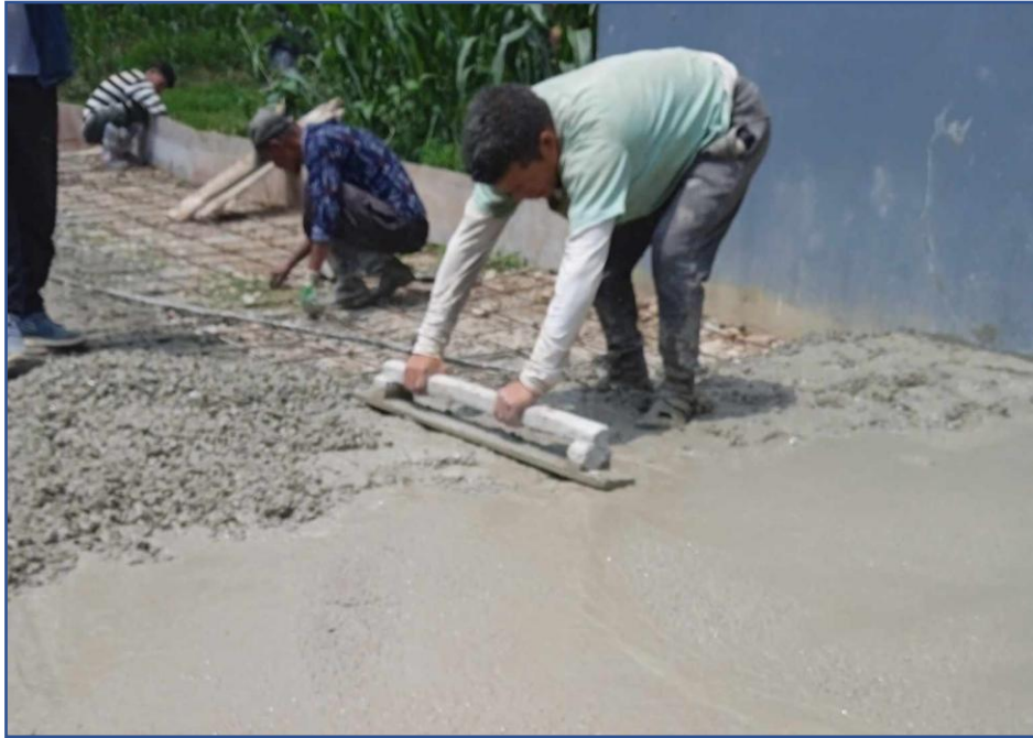
Fig : levelling surface
