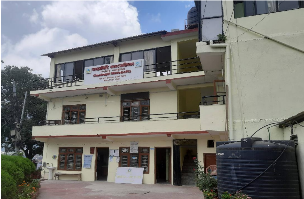
Fig : Chandragiri Municipality Ward No. 13 office
