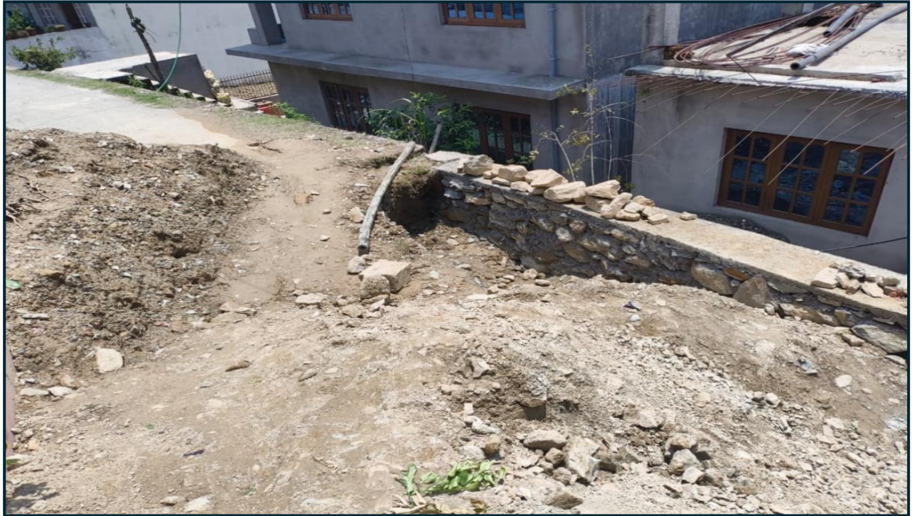
Fig: Constructed retaining wall before back filling
