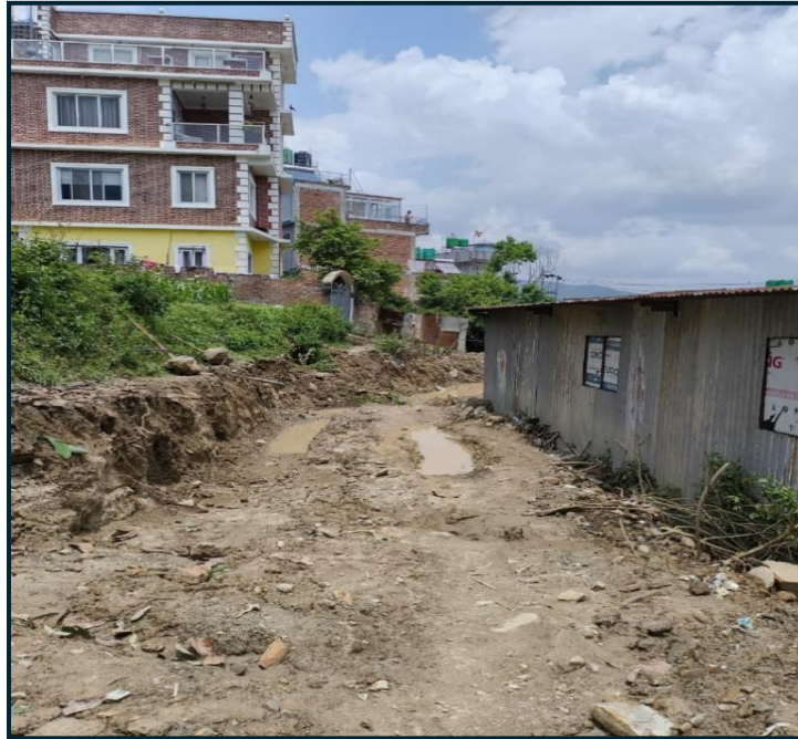
Fig: Earthen road construction
