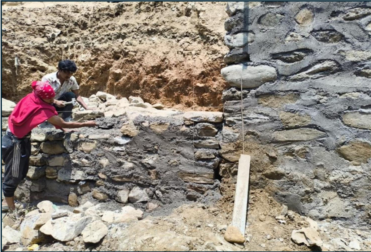
Fig: Initial stage of retaining wall before back filling
