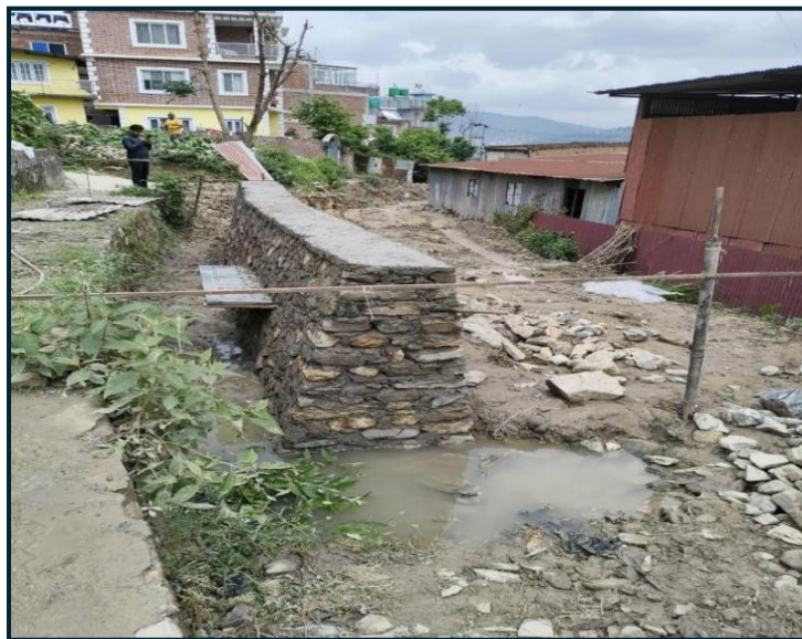
Fig: Construction of side retaining wall
